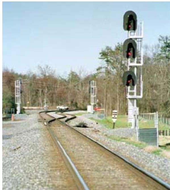
Figure 11: Control Point with Three Signal Heads
