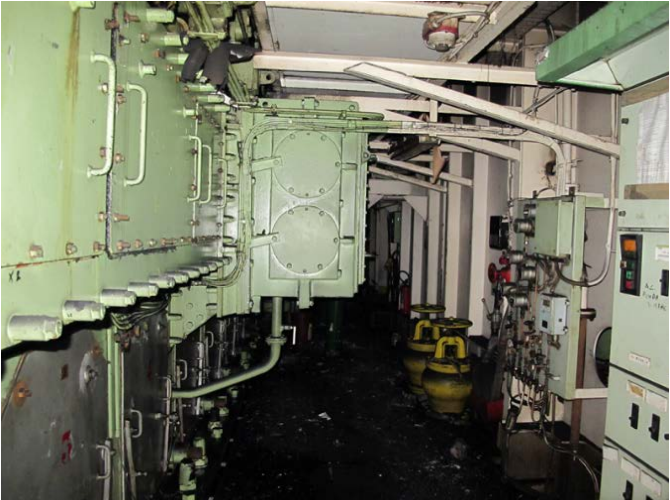
Figure 29. Photograph of portion of lower engine room.
