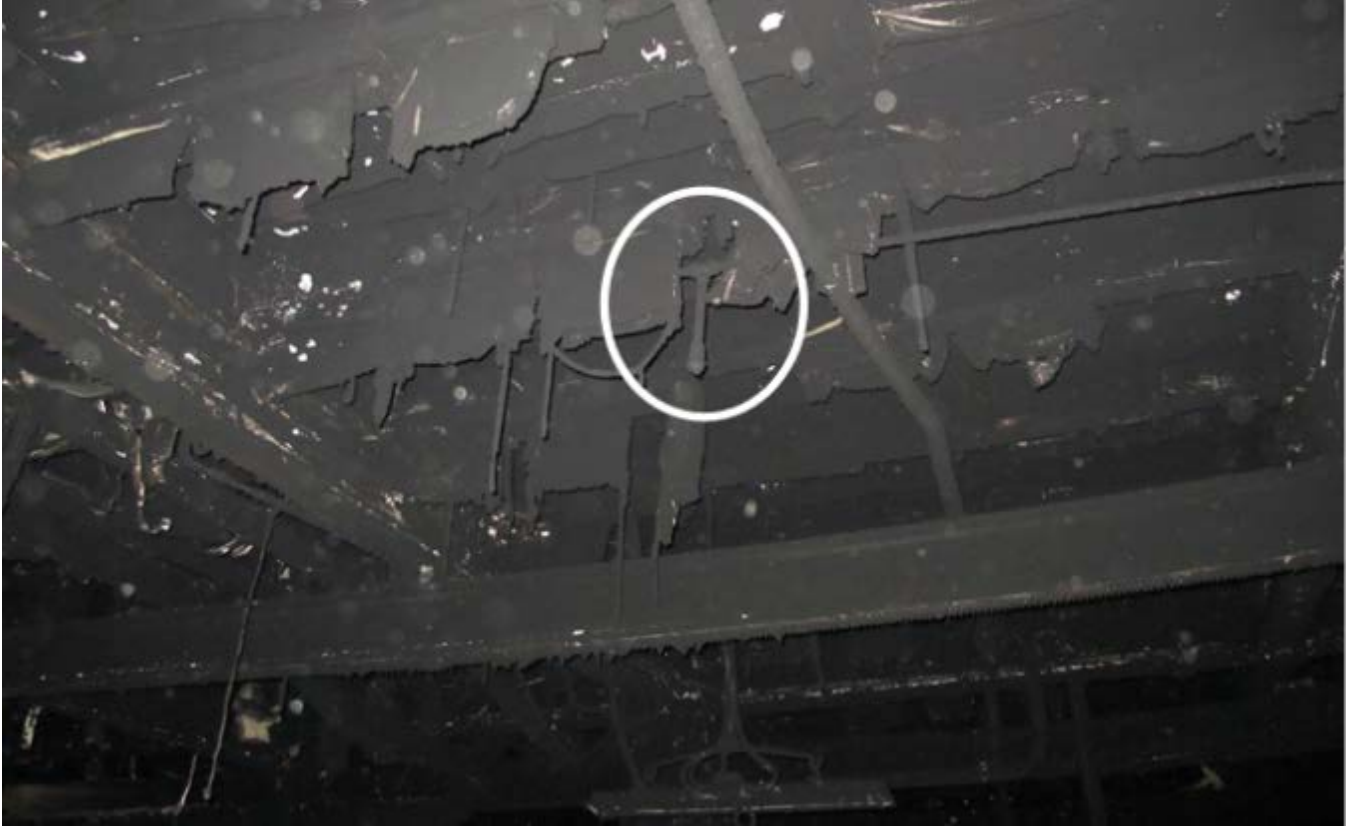
Figure 17. Photograph of water mist system nozzle after the fire. The nozzle is circled.
