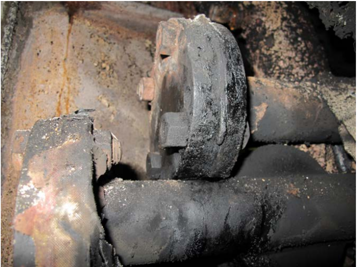
Figure 31. Photograph of flange on fuel supply line for portside main engine.
