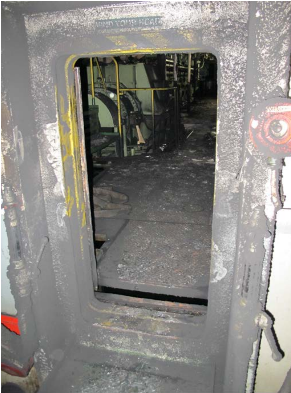
Figure 30. Photograph of watertight door 6 (facing aft into auxiliary engine room).
