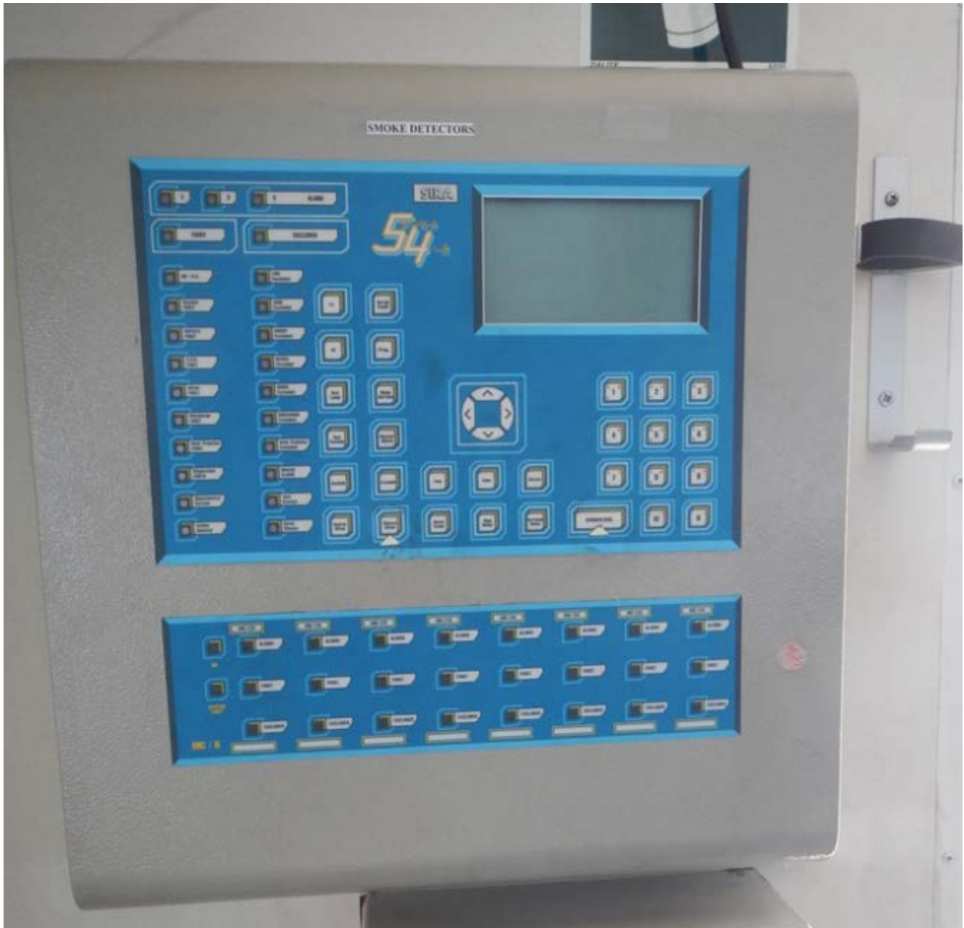
Figure 7. Photograph of SIRA panel located on the bridge.
