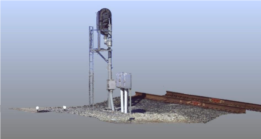
Figure 21: An image from the 3D laser scanner point cloud showing the back side of the signal.
