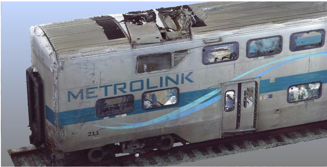
Figure 9: An image from the 3D laser scanner point cloud showing the roof damage from the left side of the 3 rd rail car - 211. (The A end is on the left side of the image.)
