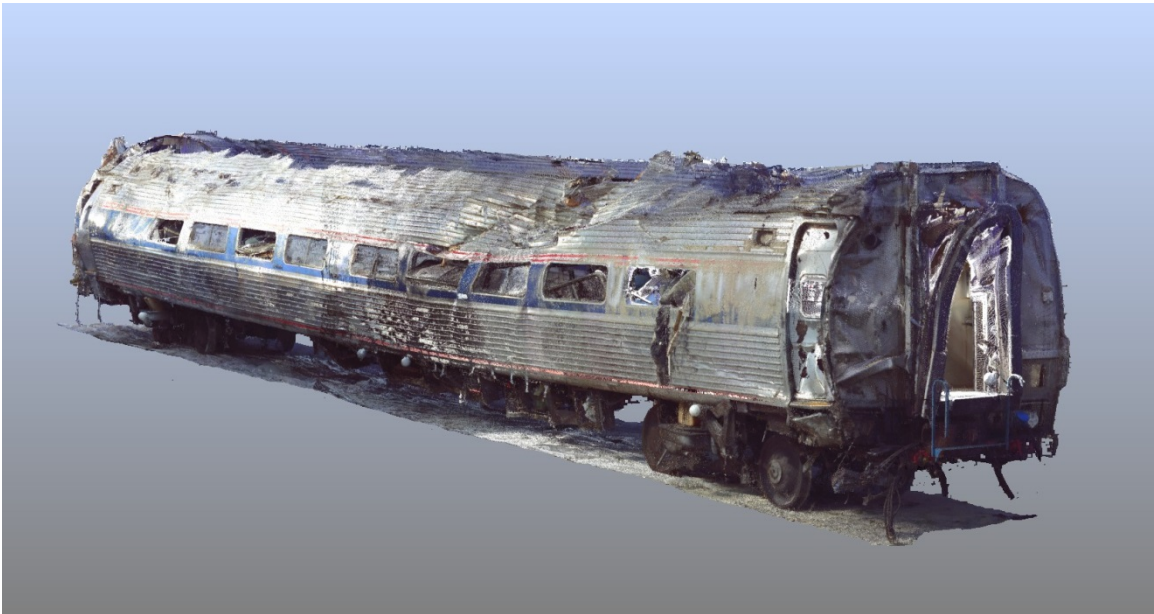
Figure 13. An image from the 3D laser scanner point cloud showing the B-end of passenger Car 2 from the other side.
