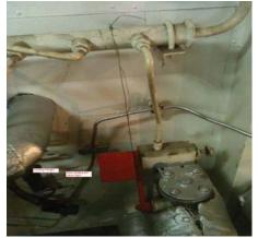
QCV blocked utilizing a bolt to hold in the open position. (Note: the painted portion on the bolt indicating possible long term condition.)
