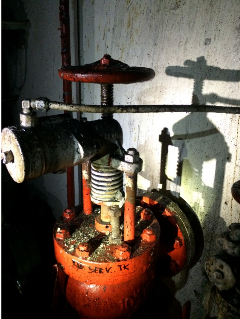
Figure 11. Caribbean Fantasy's port MGO service tank QCV that was intentionally blocked open with a bolt and nut.
