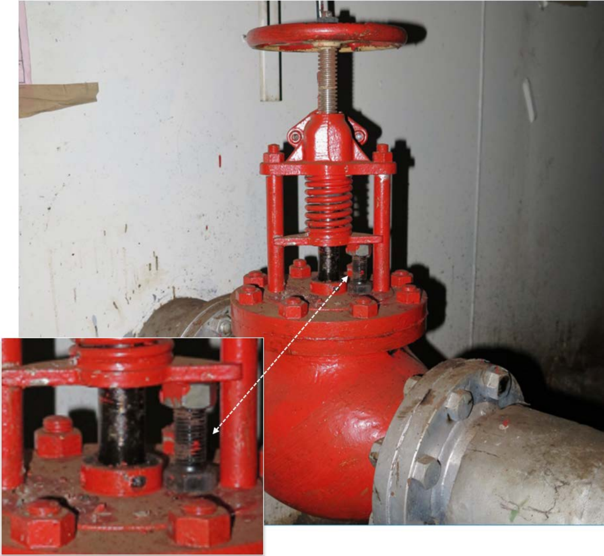
1 2 Figure 12. Caribbean Fantasy's starboard HFO storage tank QCV that was intentionally blocked open 3 with a bolt and nut. Lower left image of close up view of the bolt and nut with paint and dust.
