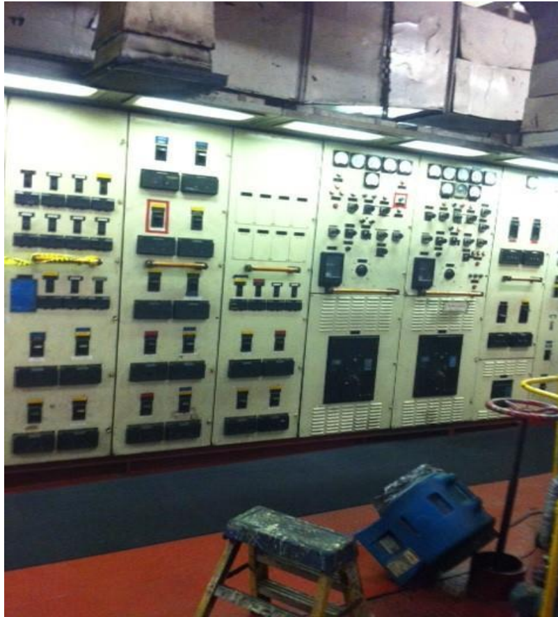
2 Figure 6. El Faro's main 450-volt electrical switchboard (photo by Maine Maritime Academy cadet).
