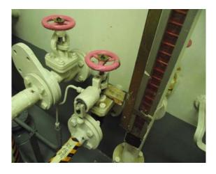
QCV blocked utilizing a wooden block to hold the valve in the open position.
