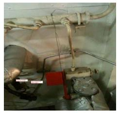
QCV blocked utilizing wire to hold closing weight up and the valve in the open position.
