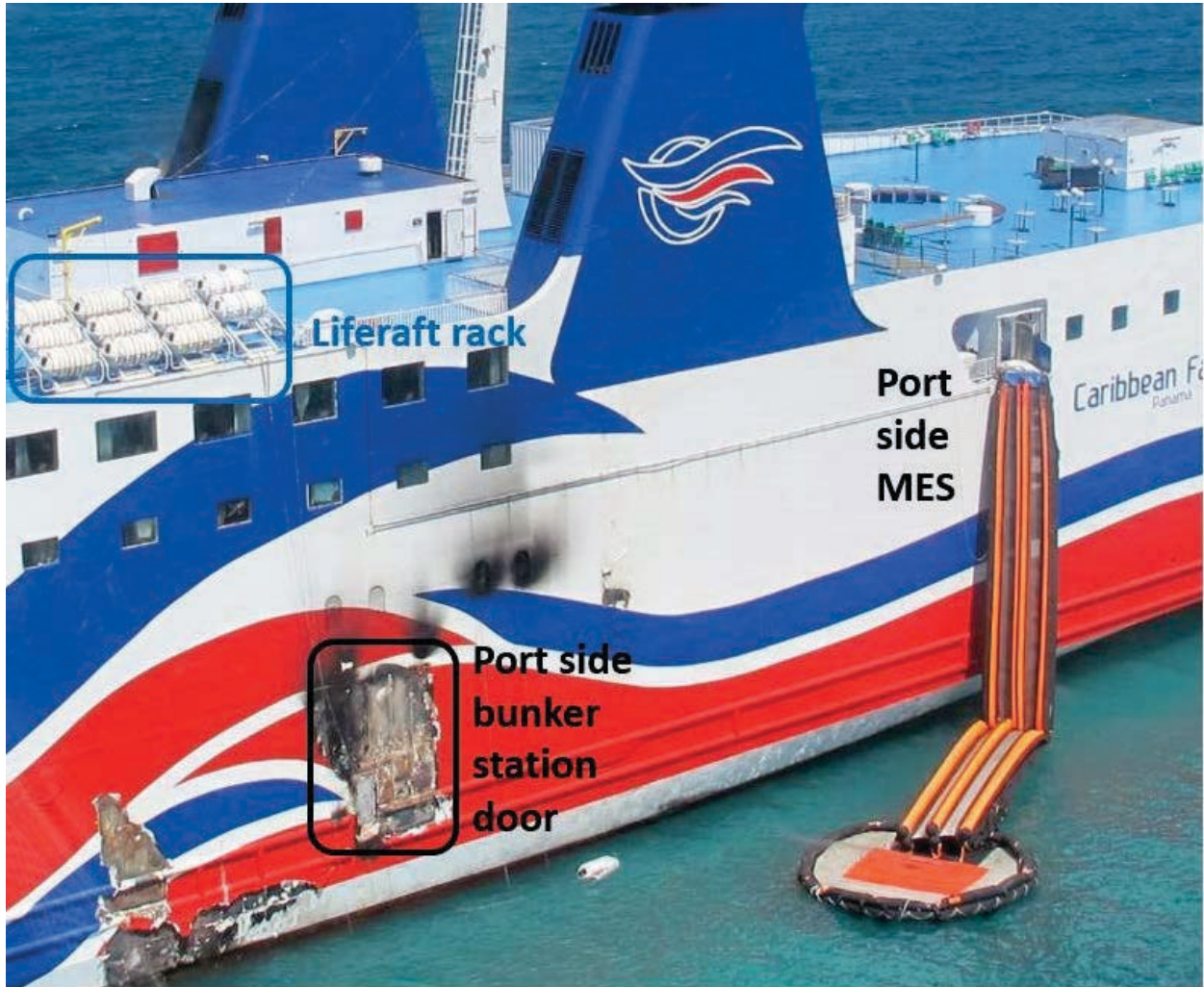
7 8 Figure 9. Aerial photograph of the port side of the Caribbean Fantasy taken on August 9 19. A black rectangle highlights the location of the port side bunker station shell door. 10 Note the burned paint in the surrounding area and the soot stains around some of the 11 ventilation louvers. A blue rectangle outlines the main rack housing the 12 liferafts. All 12 rafts remain in the rack except for one, which floats uninflated in the water. Also note the 13 steep angle of the MES slide.
