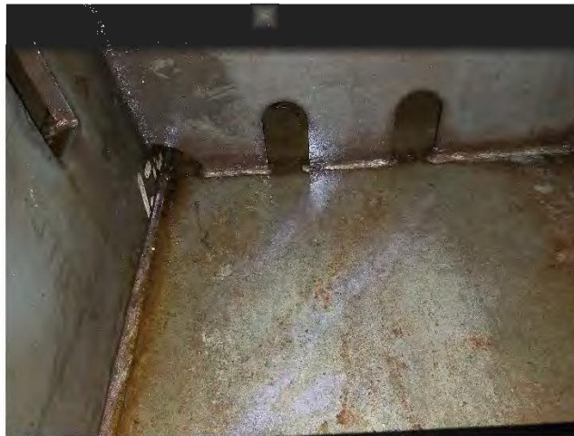
Limber Holes Port Side/ Center Channel/ After Bay Looking Forward
