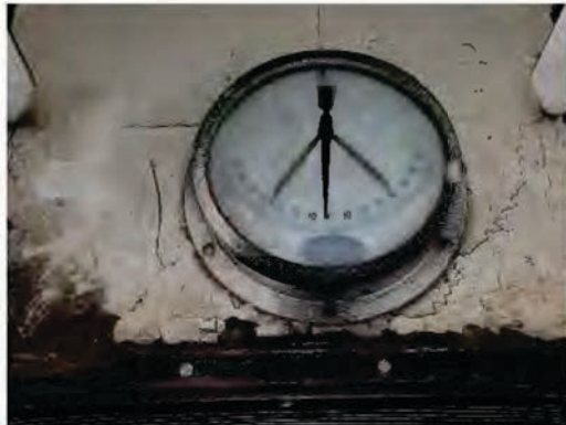
Clinometer Mounted in Engine Room Operating Platform
