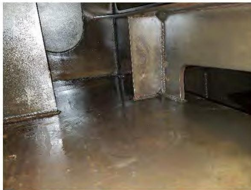
Main Engine Lube Oil Sump from Inner Bottom Level Port Side
