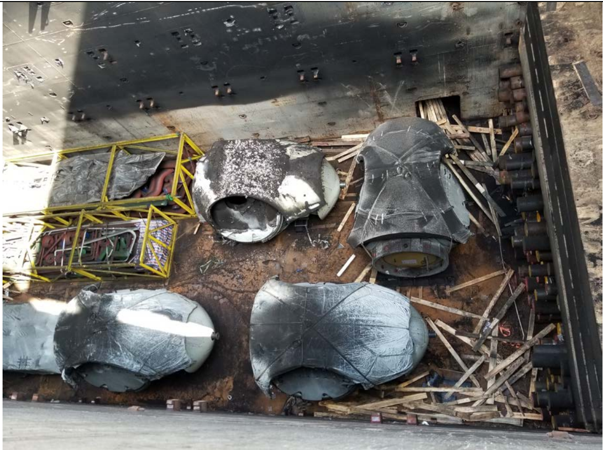
View into fire affected lower cargo hold #3 port side; burnt hub #18020106 in upper left corner of picture
