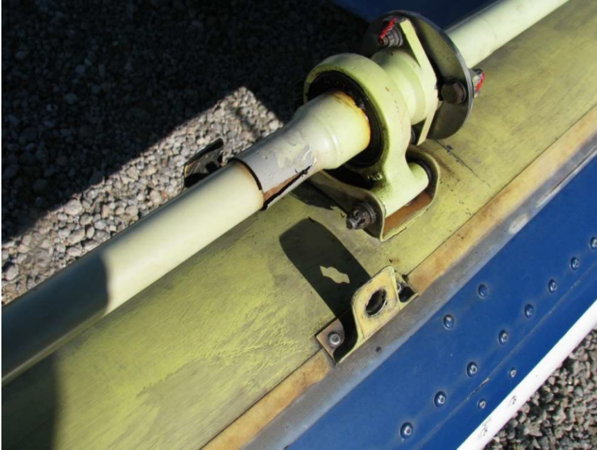
Figure 1: The separated splined adapter at the forward end of the No. 4 segmented tail rotor drive shaft. Photo courtesy of Bell Helicopters.
