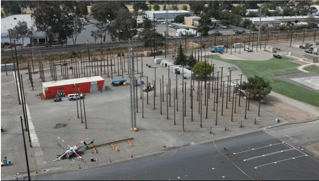
Figure 2 - Accident location within training facility (photo courtesy of PG&E).
